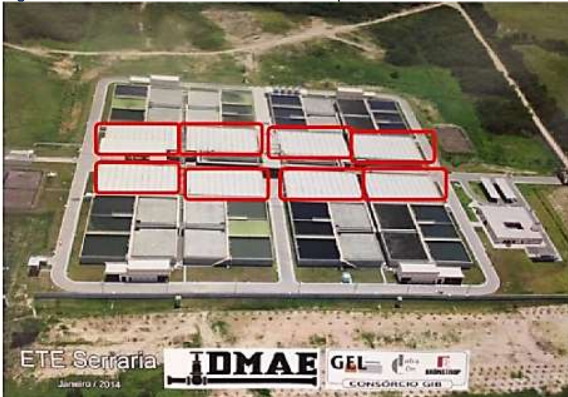
Figure 5 - Panoramic view of STP Serraria with emphasis on UASBs
